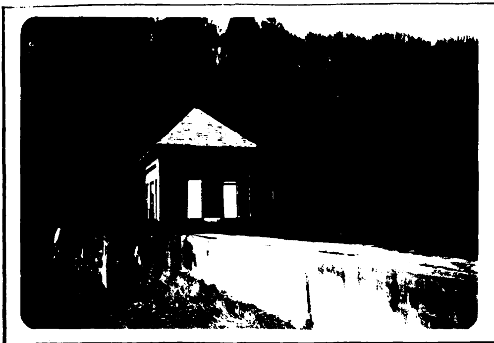
1. CREST OF DAM SHOWING GATE HOUSE, HOIST PLATFORM AND HOIST, AND CONCRETE WALL. (12/3/80)
