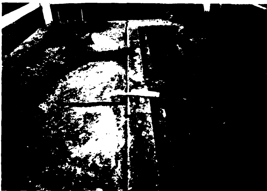
Photo # 6 Deteriorated concrete at roof of right spillway structure (rule extended 1 ft.)
