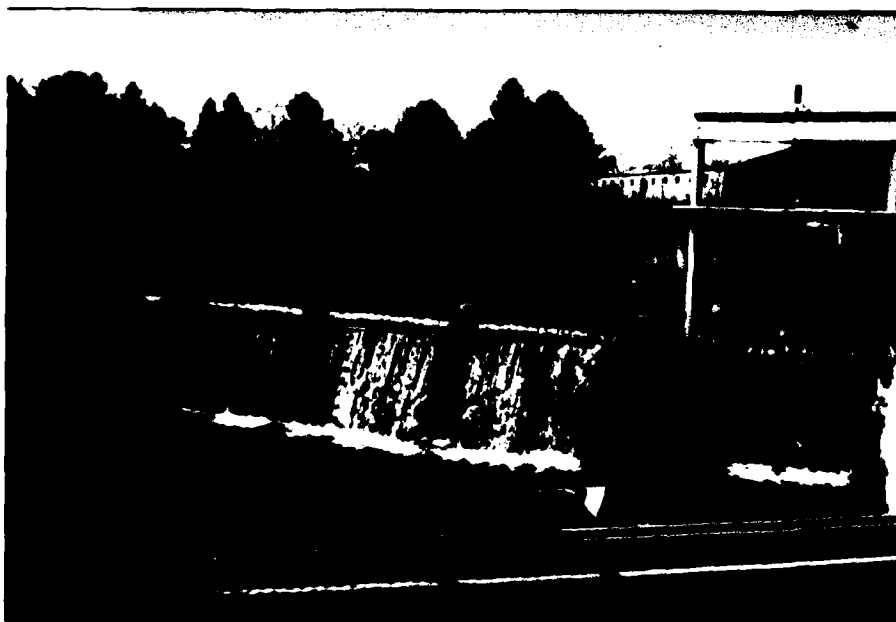
NO. 2 SHARP CRESTED WEIR AND LOW LEVEL GATE
