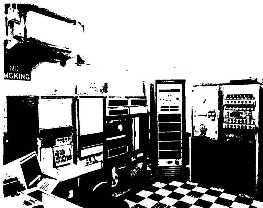
Fig. 7 - Computer Control System
