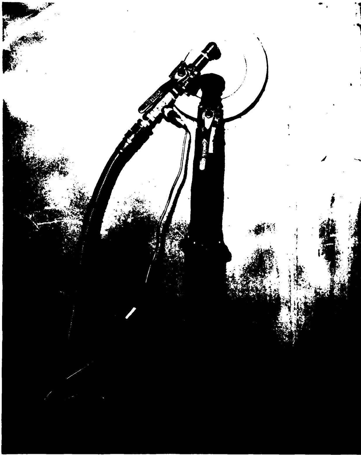
FIGURE 6. Flow Meter installed externally on an aluminum two-lock chamber.
