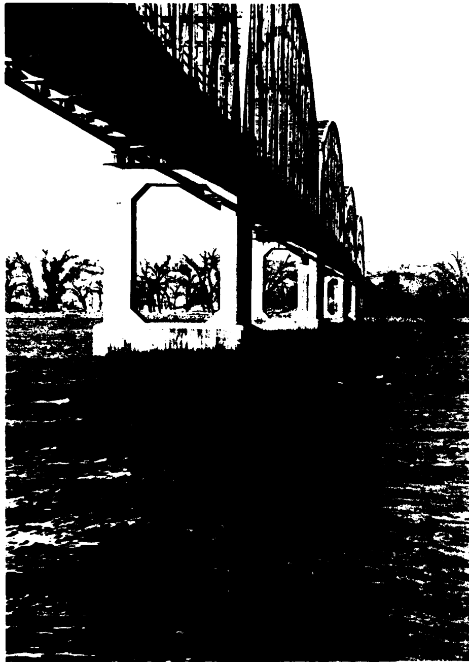
Figure 0-10. Old U. S. Highway 14 Bridge over the Missouri River at Pierre, South Dakota. View showing the river piers, looking west. Photo: D. Murphy.
