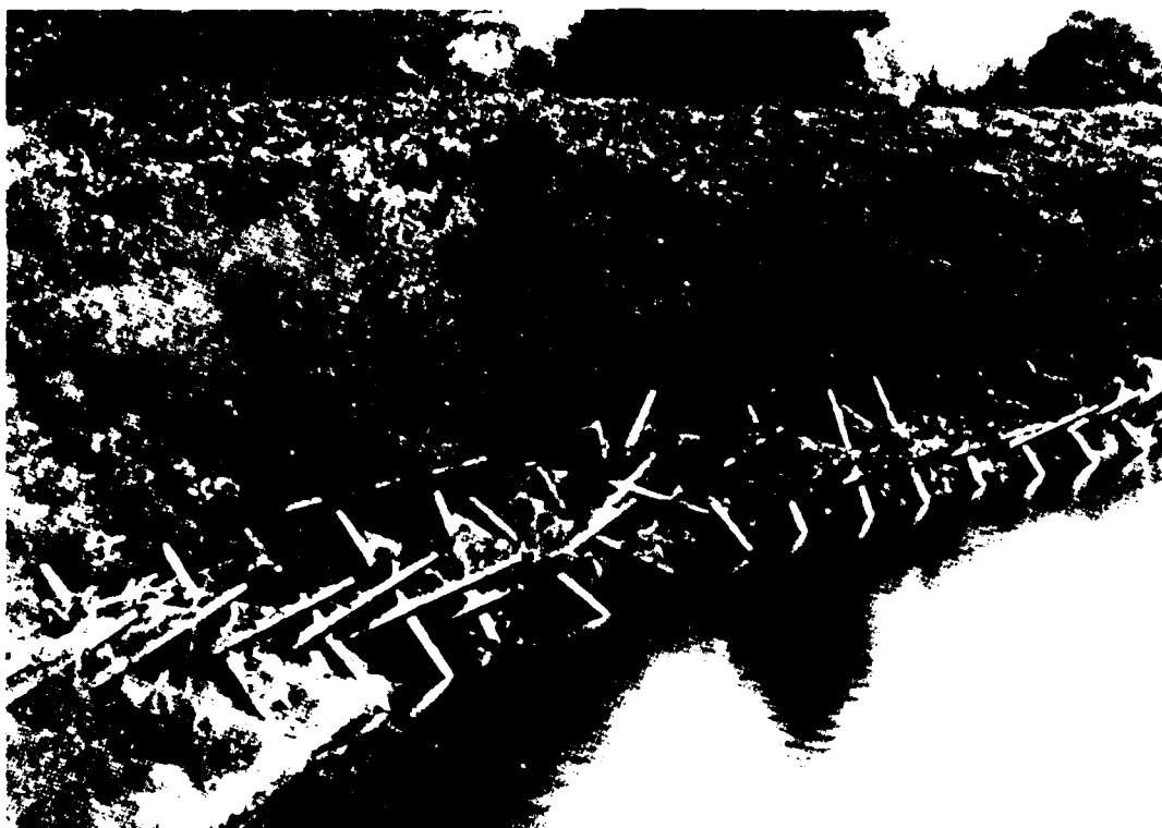
Figure 42. Kellner jacks placed longitudinally along the bank; note vegetation behind the jack line (photo courtesy of SCS)
