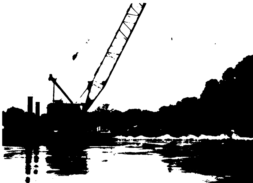
Figure 49. Floating plant construction
