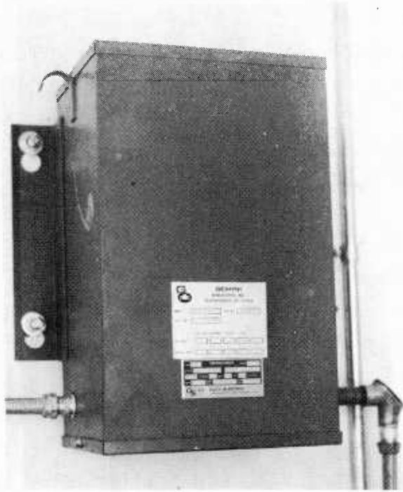
FIGURE 2-14. Typical Isolation Transformer.
