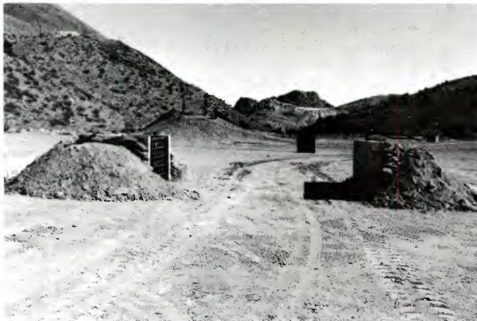
VIEW SHOWING REVETMENT WALL - BEFORE TEST
