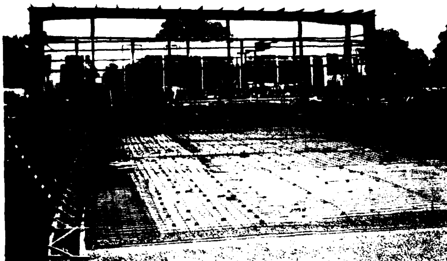
Figure 9. Rigid-frame, clear-span structure for natatorium--Fort Benjamin Harrison.
