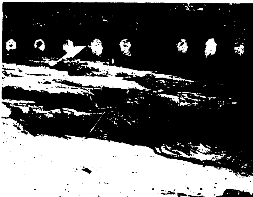
31. Harry S. Truman Dam, 11 November 1966, Neg. No. R-262-8. Cutoff Trench Sta. 23+00 looking upstation. Caves on downstream side Sta. 23+40 to Sta. 23+80.
