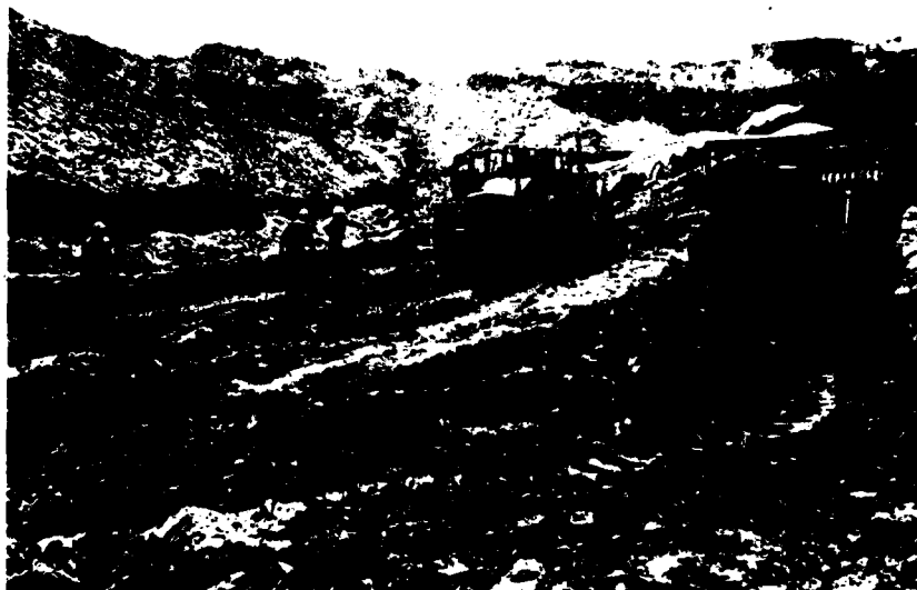
7. Harry S. Truman Dam, 27 July 1966, Neg. No. R-245-9. Cutoff Trench Sta. 51+15. Looking downstation placing pervious and impervious fill.
