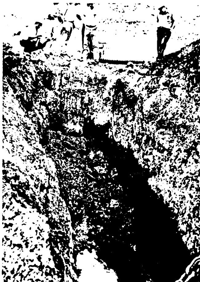
195. Harry S. Truman Dam, 22 September 1977, Neg. No. 77-534. Dewatering trench in basal gravel before installation of collector pipe.
