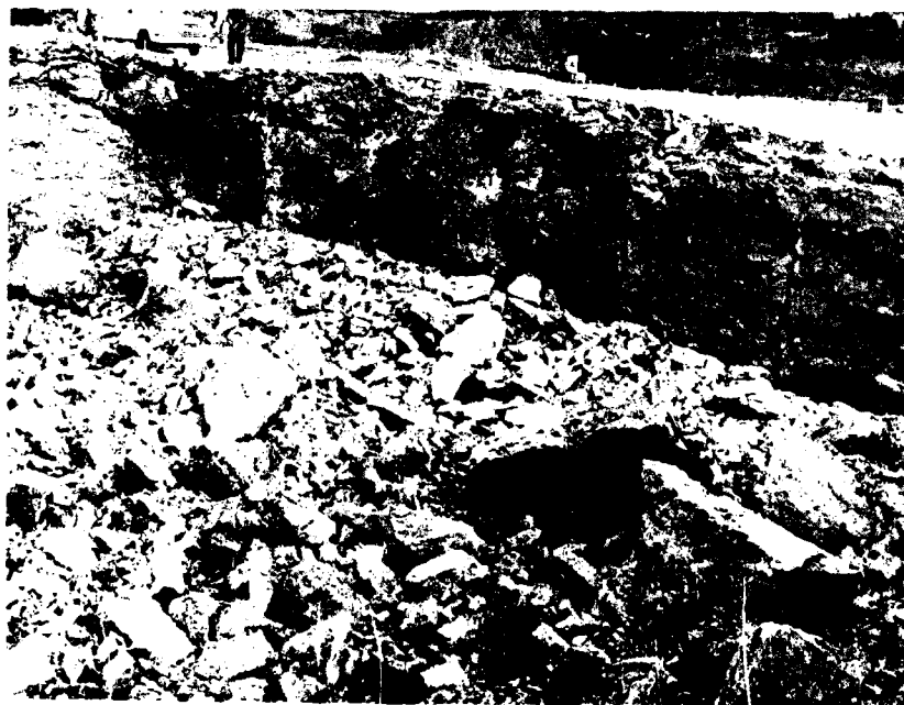
42. Harry S. Truman Dam, 28 October 1966, Neg. No. 82737. Spillway-Powerhouse excavation. Experimental blasting.
