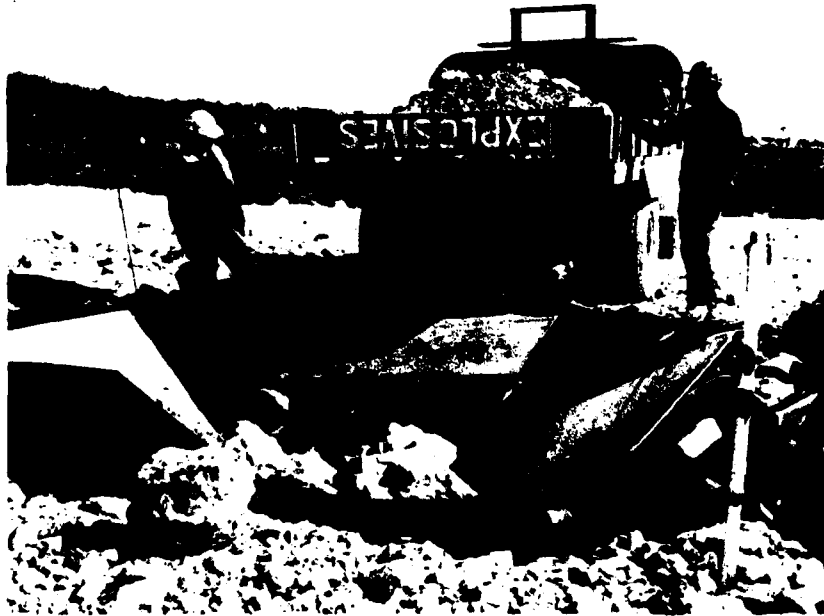
B-1. End dumping sample into hole. 23 March 1968, Neg. No. 85141.
