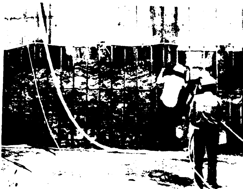
104. Harry S. Truman Dam, 28 April 1972, Neg. No. 965-35. Spillway-Powerhouse. Monolith 5, right wall. Ready for concrete pour 3c.
