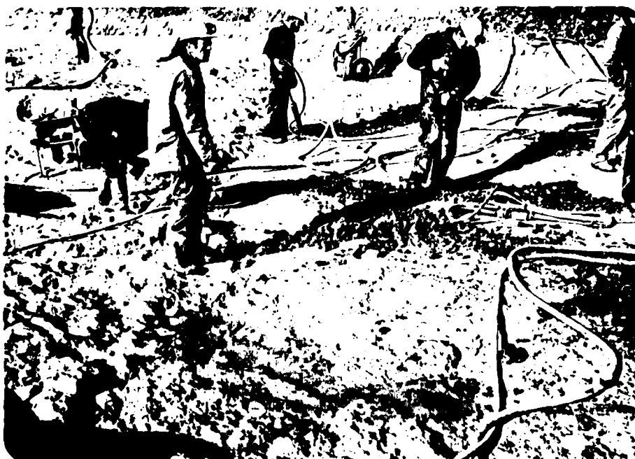
207. Harry S. Truman Dam, 25 November 1977, Neg. No. 77-718. Closure area cutoff trench, Sta. 63+50. Placing impervious clay in open joints.
