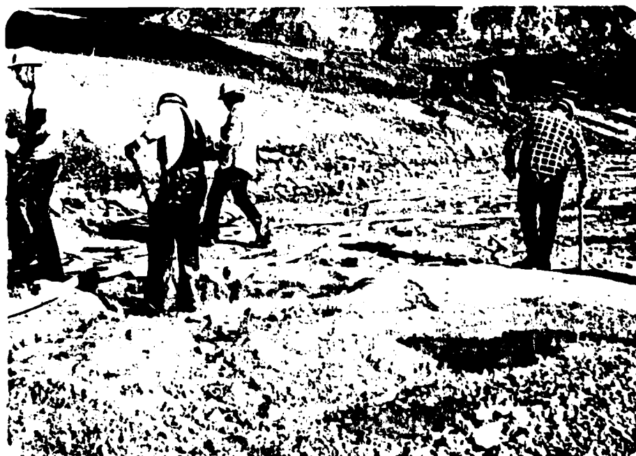
203. Harry S. Truman Dam, 11 November 1977, Neg. No. 77-668. Closure area Sta. 62+90 cutoff trench. Cleaning foundation surface.
