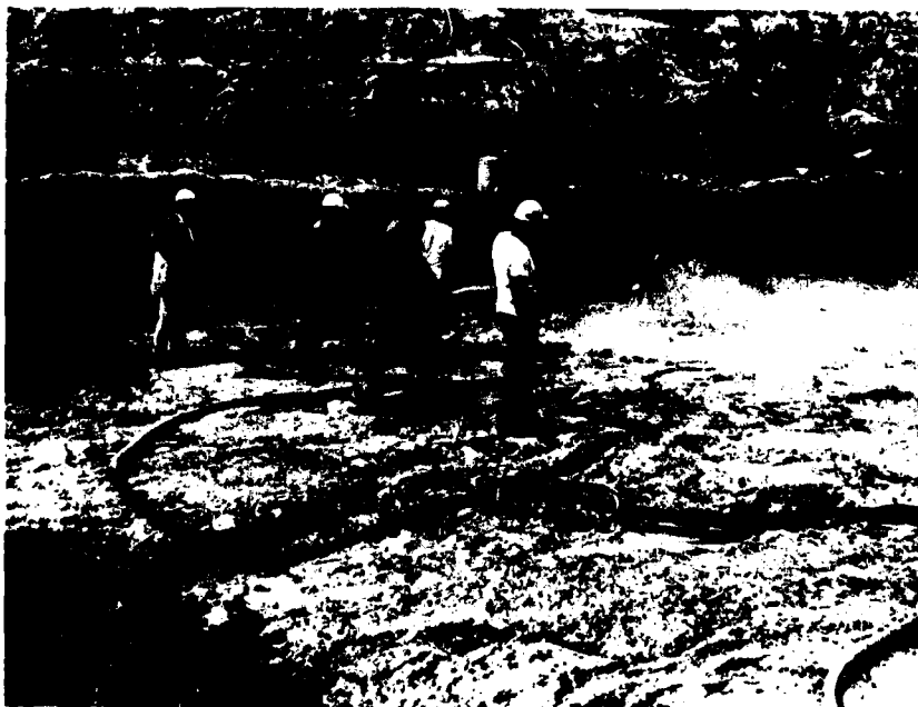
8. Harry S. Truman Dam, 27 July 1966, Neg. No. R-245-12. Cutoff Trench Sta. 51+90. Looking upstream. Foundation cleanup.
