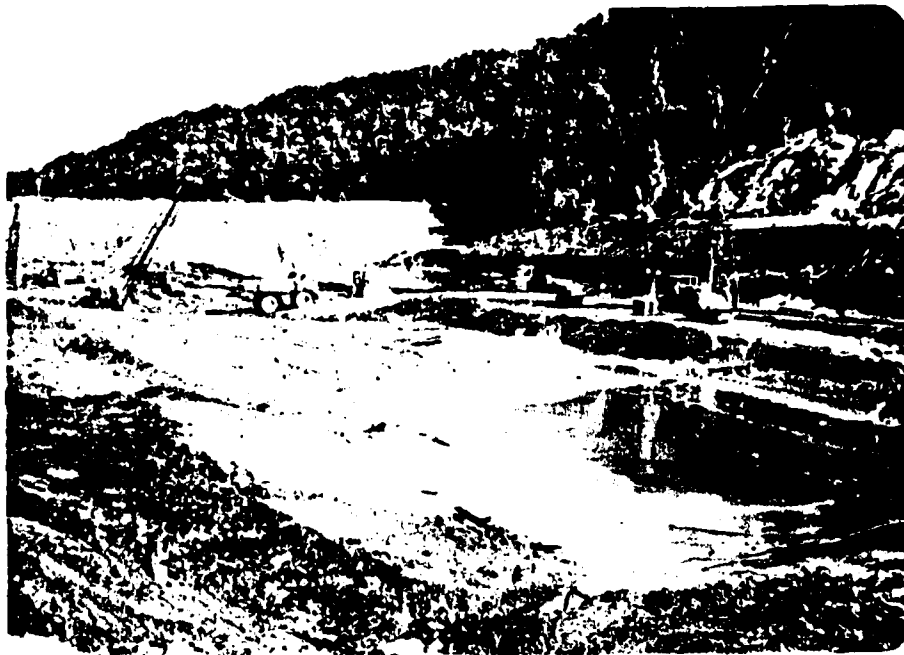
185. Harry S. Truman Dam, 29 July 1977, Neg. No. 77-429. Closure area. Excavating muck. Looking upstream.
