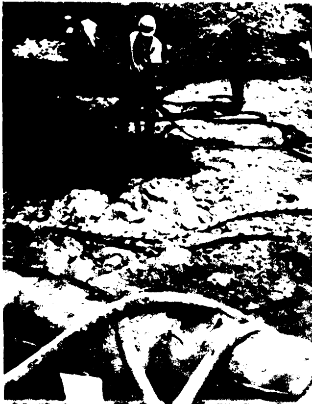
215. Harry S. Truman Dam, 30 May 1978, Neg. No. 965-112. Closure area cutoff trench Sta. 69+50. Hand tamping impervious clay on breccia bedrock surface.
