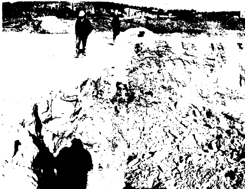
41. Harry S. Truman Dam, 28 October 1966, Neg. No. 82734. Spillway-Powerhouse excavation. Experimental blasting.
