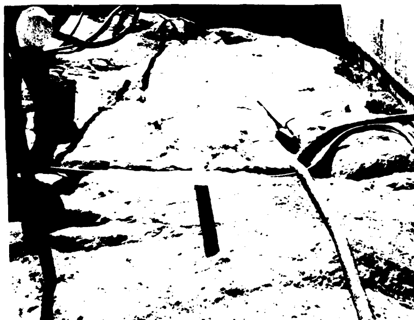
82. Harry S. Truman Dam, 23 March 1972, Neg. No. R-965-116 Spillway-Powerhouse. Rock Surface to receive backfill concrete along downstream wall of Monolith 3 looking right.
