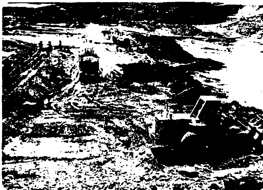
186. Harry S. Truman Dam, 2 September 1977, Neg. No. 77-502. Muck excavation, closure area. Looking upstream at Sta. 69+50.
