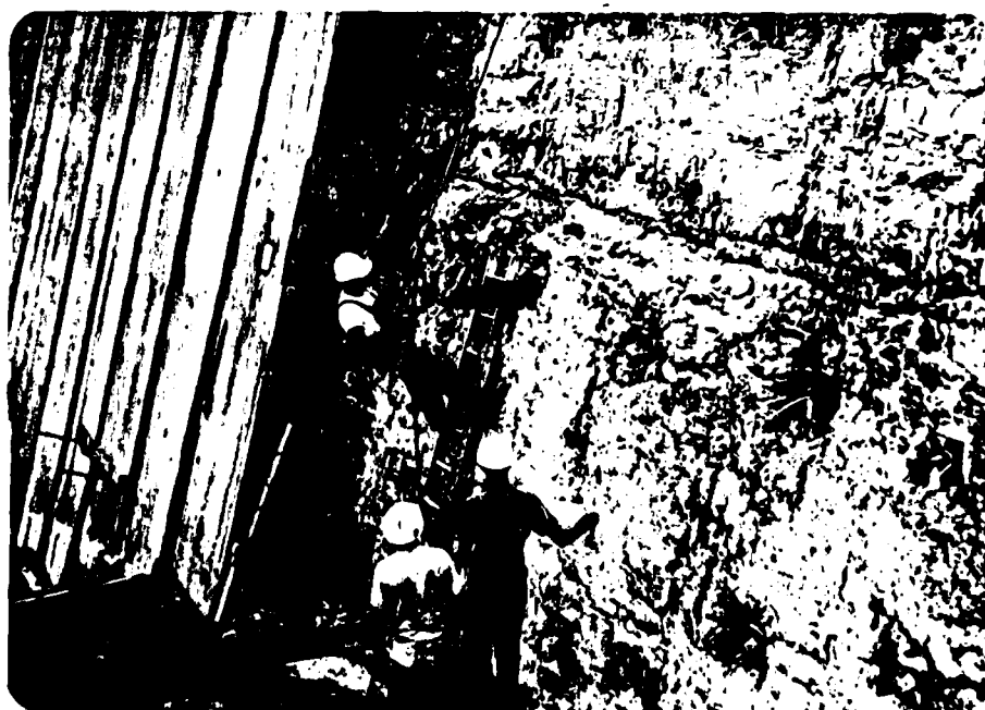
236. Harry S. Truman Dam, 2 July 1973, Neg. No. 73-272. Pull out test on rock bolts.
