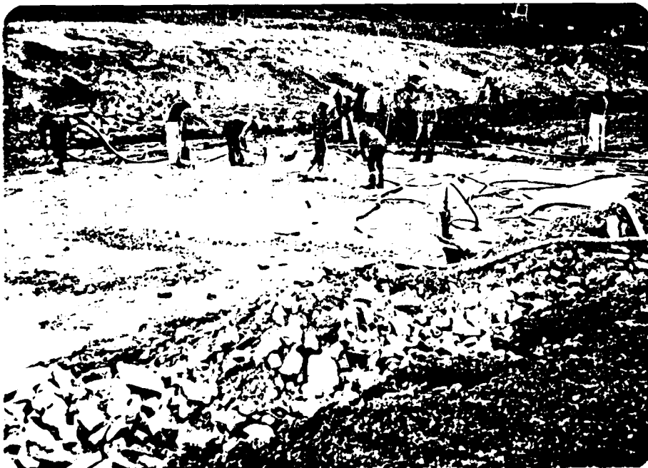
206. Harry S. Truman Dam, 11 November 1977, Neg. No. 77-702. Closure area cutoff trench, Sta. 63+10. Cleaning foundation surface.
