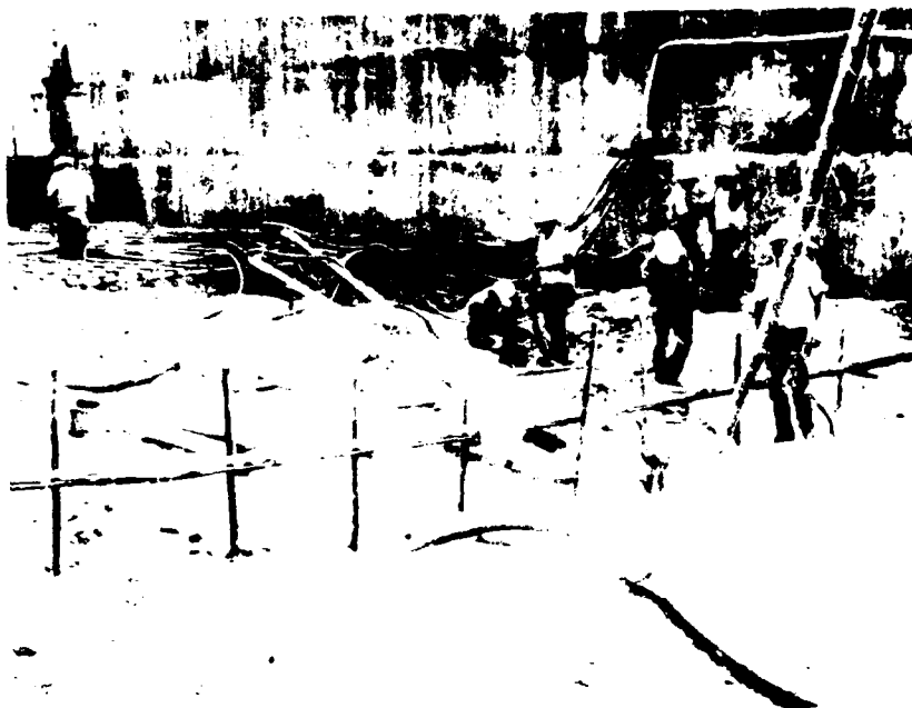
113. Harry S. Truman Dam, 7 June 1972, Neg. No. 965-62. Spillway-Powerhouse. Foundation Monolith 12. Looking downstream. Ready for concrete lift 3.
