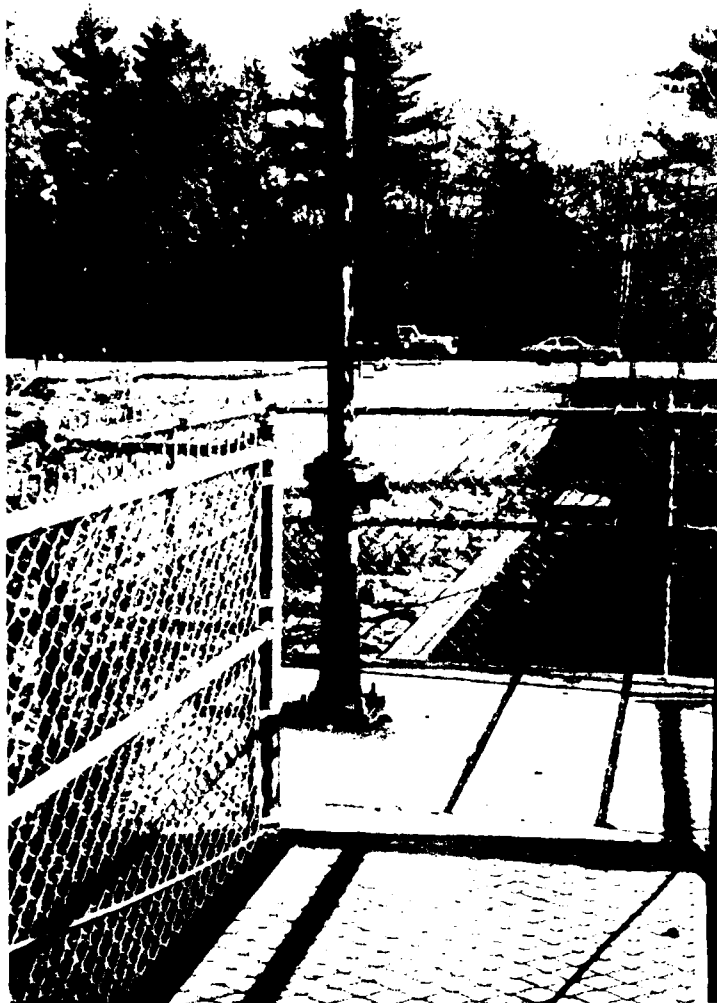
10. VIEW OF LOW LEVEL GATE OPERATING STAND.
