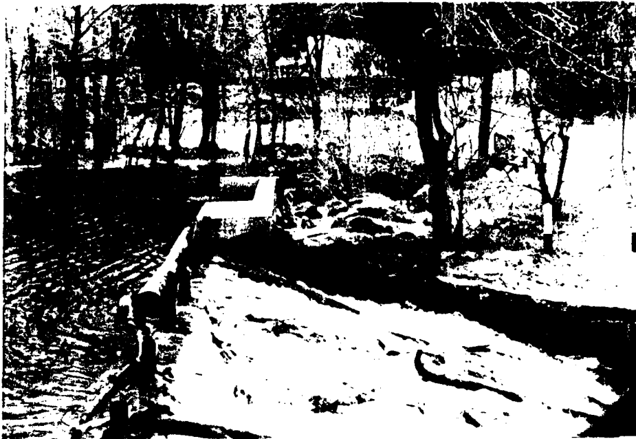
13. Concrete wall separating two spillways
