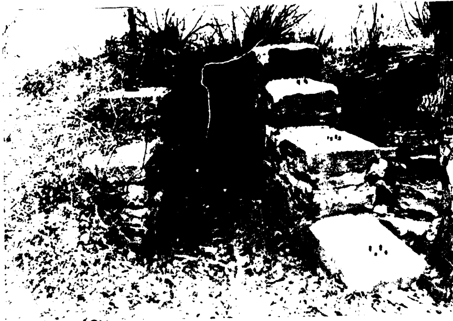
17. Sluice gate outlet in earth embankment blocked by concrete
