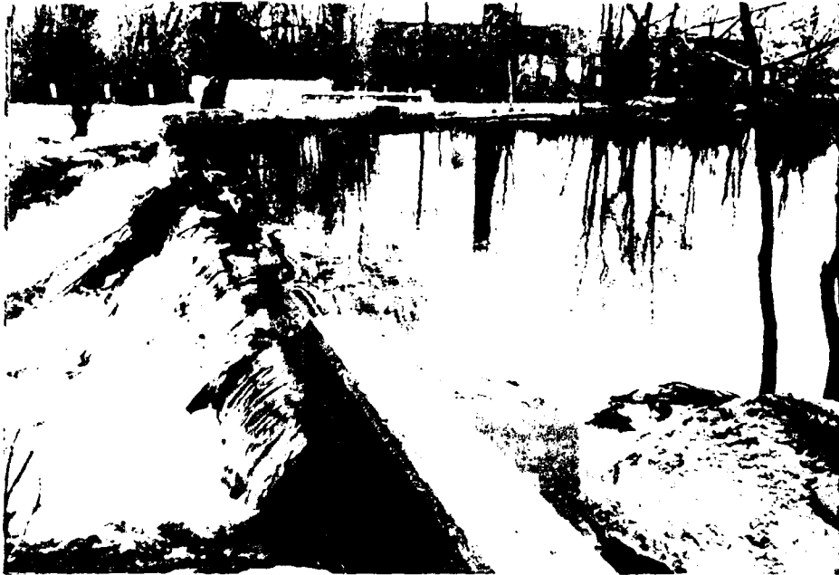
15. Weir and trapped debris at left (northerly) spillway
