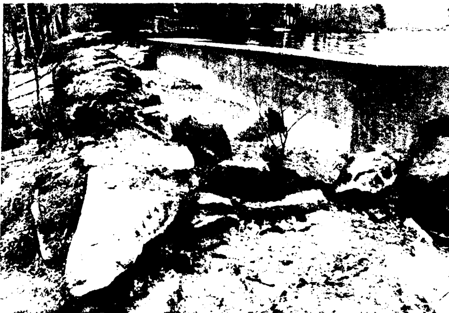
14. Eroded earth berm on downstream side of concrete wall
