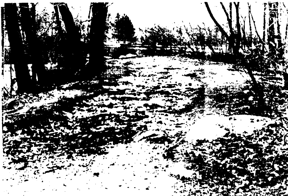
10. Badly eroded unpaved road at left abutment of dam
