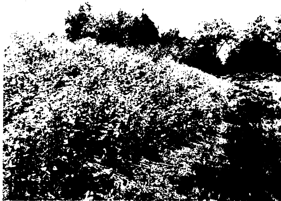
2. Brush growth along downstream slope of main dam.
