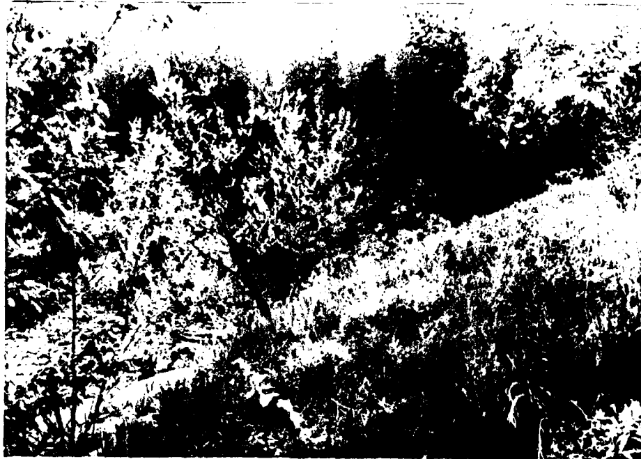
7. Brush and tree growth on upstream slope of Dike A.
