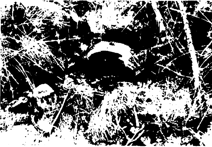
Photo #6 View of upstream end of culvert under Navin Rd. looking southerly from toe of dike. Note culvert 2/3 plugged
