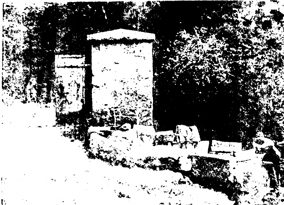
4. Left side of gate structure
