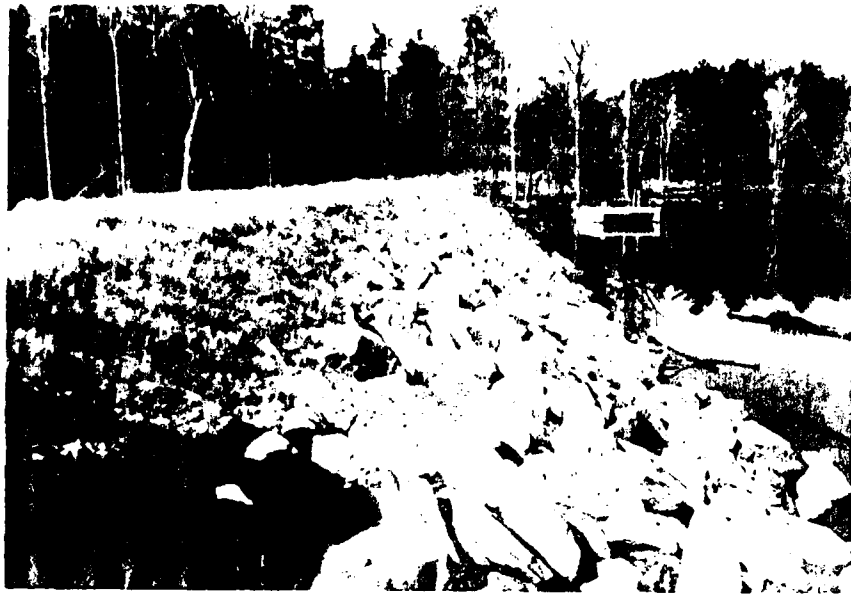
Photo 1 - Dam overview looking westerly from left abutment
