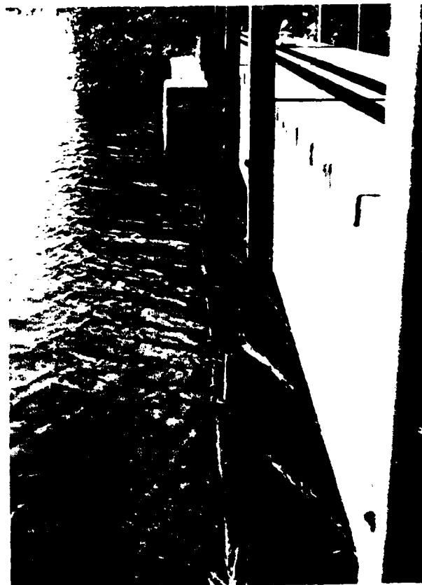
PHOTO NO.4 - Spillway flash- board assembly viewed from right side of spillway.
