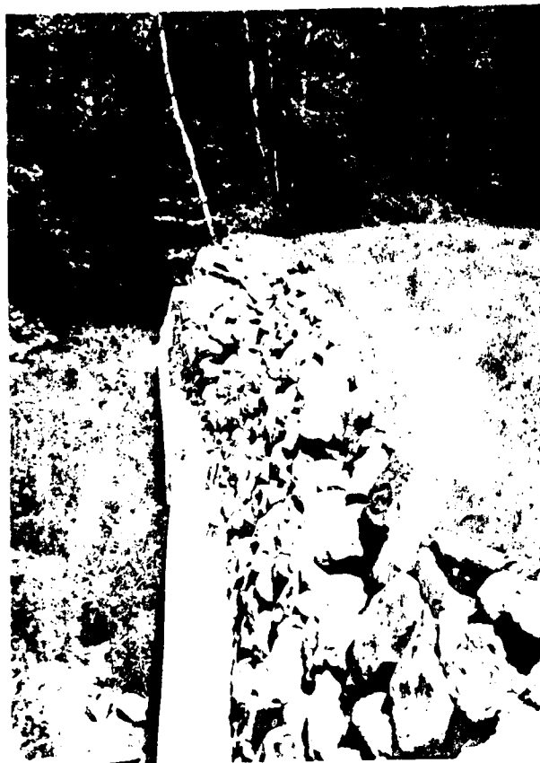
PHOTO NO.11 - Right spillway training wall showing wall misalignments and movements and subsi- dence behind the wall.
