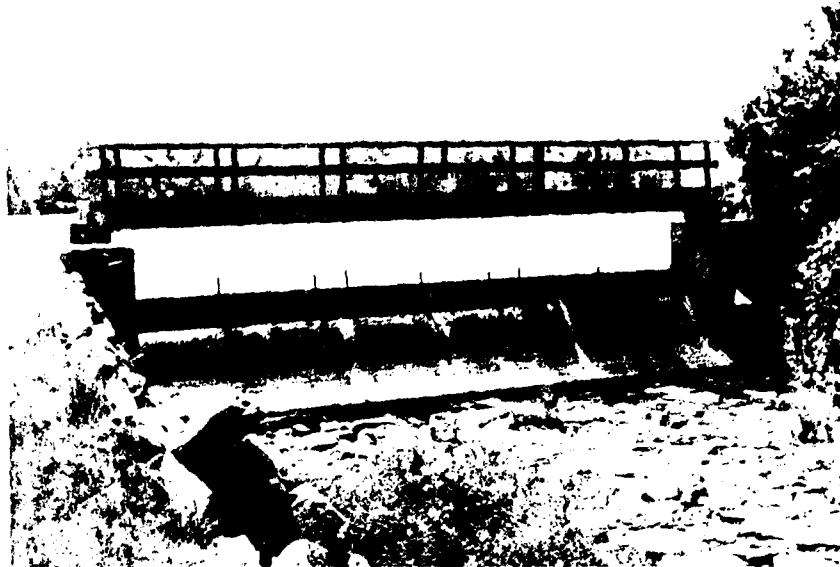
PHOTO NO.7 - View of spillway weir and bridge. There are 14 inches of flashboards in place.
