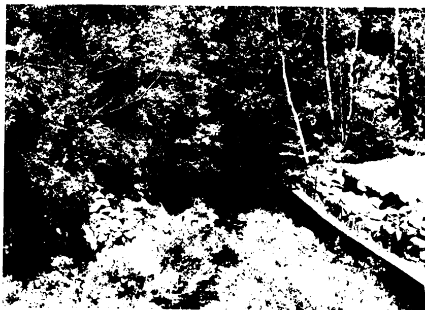
PHOTO NO.10 - General view of spillway discharge channel showing brush in channel and trees overhanging channel.
