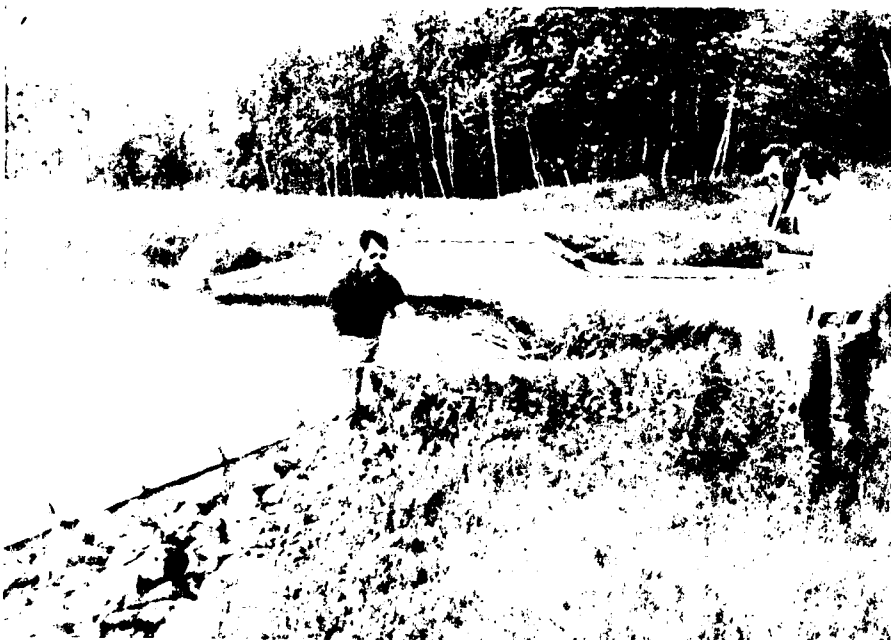
PHOTO NO. 12 - Area of subsidence of crest behind right wall of spillway below ruler in photo.
