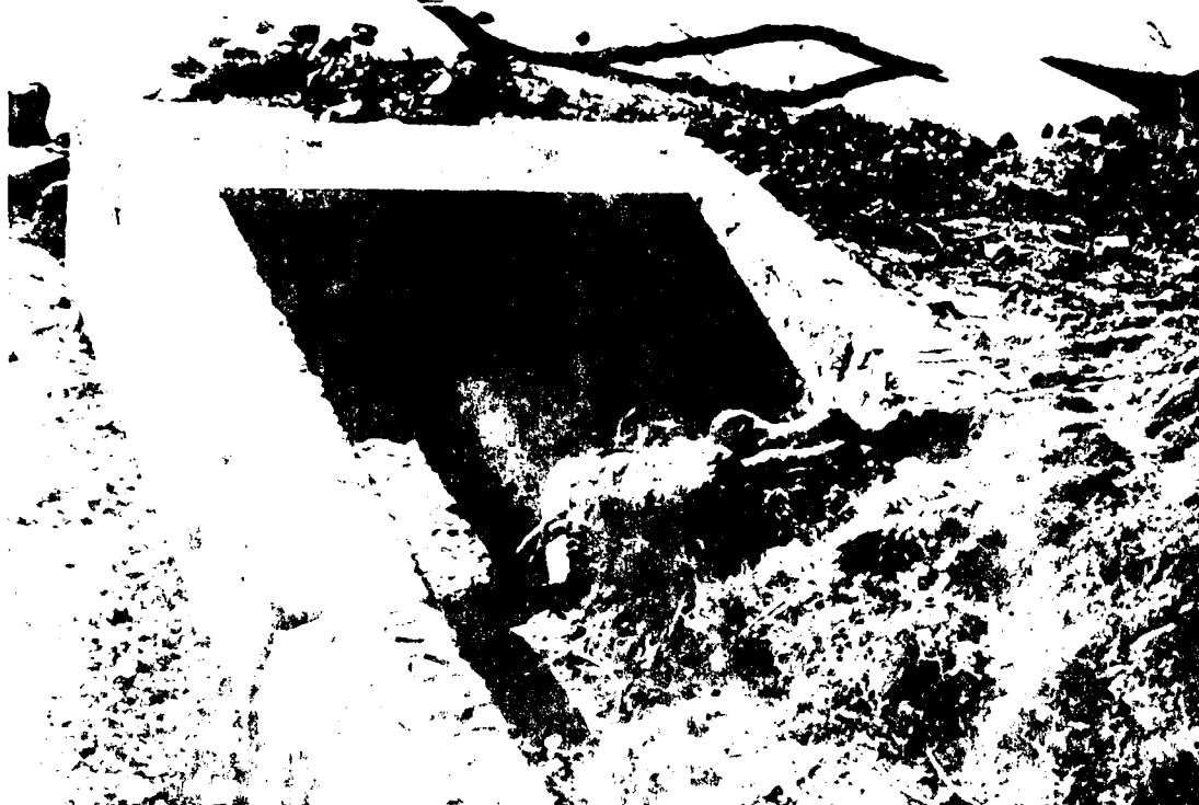
4. VIEW OF OUTLET STRUCTURE AND OUTLET PIPE. NOTE NOTCH RECENTLY CONCRETE FILLED.
