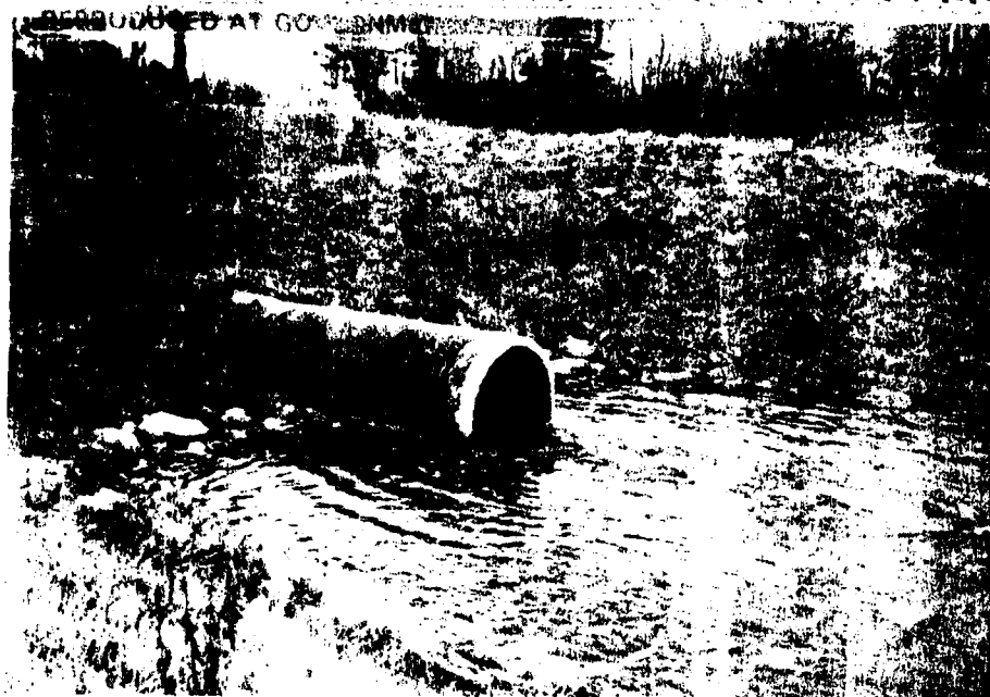
Principal spillway outlet shift at stilling basin.
