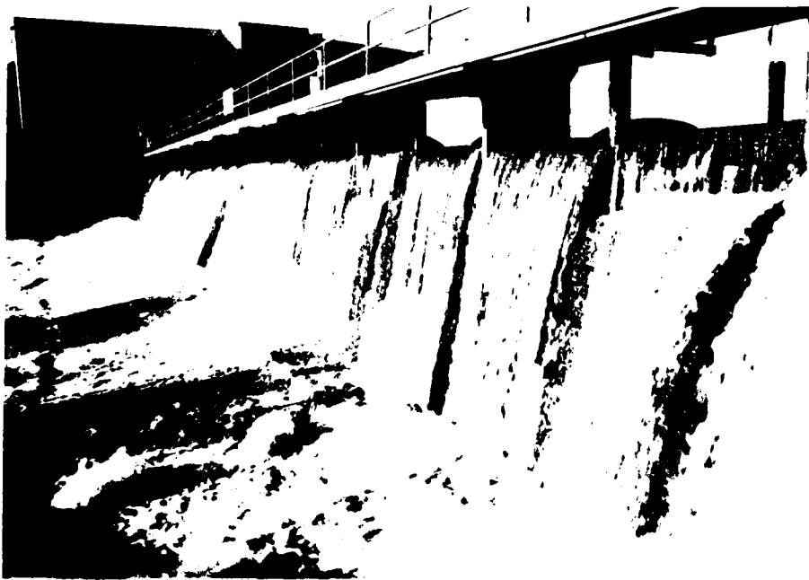
4. Spillway viewed from left bank
