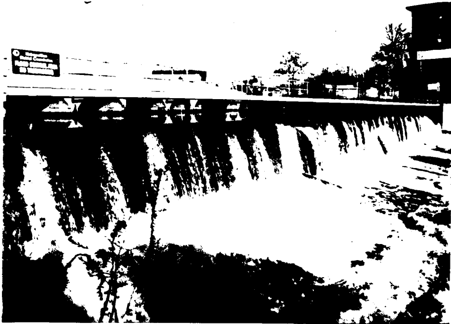
3. Spillway viewed from right bank
