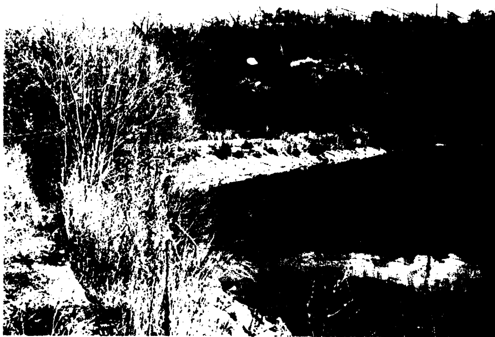
3. VIEW OF UPSTREAM SLOPE. NOTE CEMENTED STONE RIPRAP AND VEGETATION.
