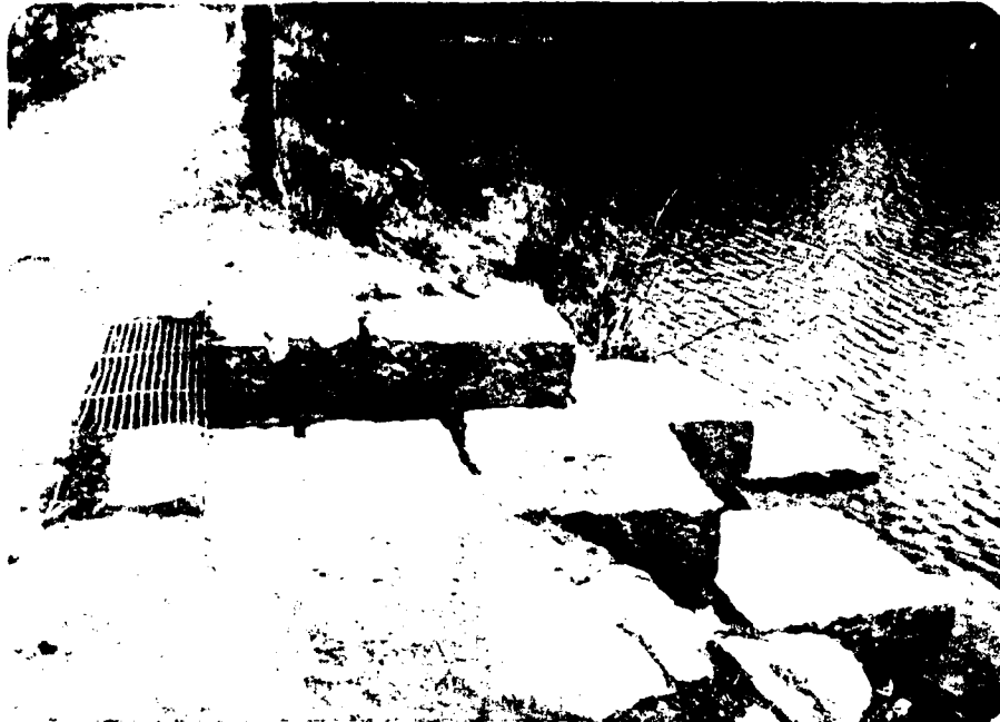
NO. 3 VIEW OF SPILLWAY
