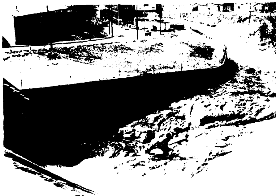
10. DOWNSTREAM CHANNEL. DISCHARGE PIPE FROM OUTLET WORKS AT END OF CONCRETE WALL LEFT SIDE OF PHOTO.
