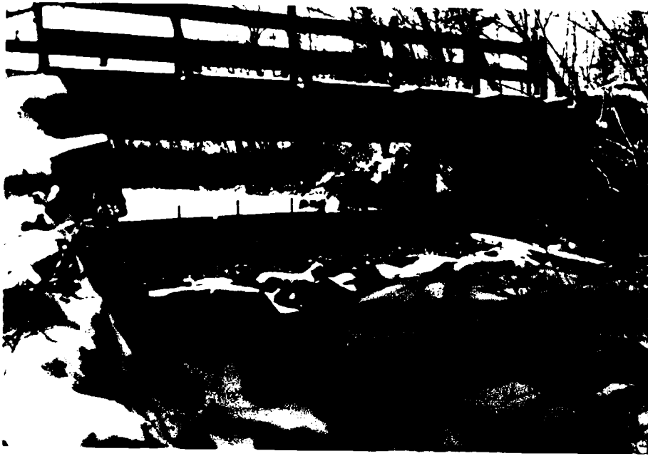
NO. 7 DOWNSTREAM VIEW OF AUXILIARY SPILLWAY WITH FLASHBOARDS
