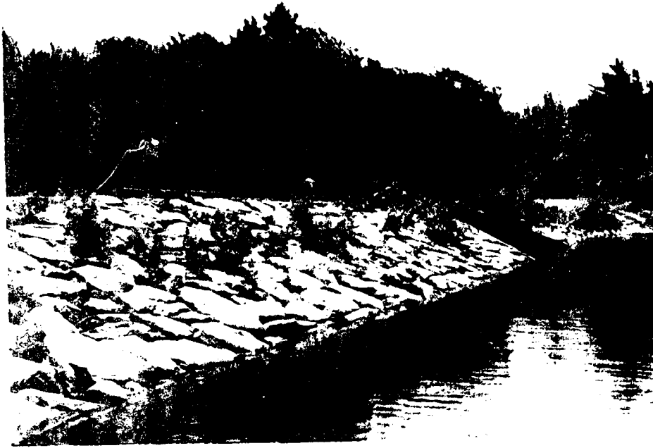
PHOTO NO. 2 - Upstream face from left abutment showing riprap and small brush.
