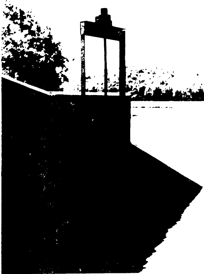
PHOTO NO. 6 - View of manually controlled gate for main drain.
