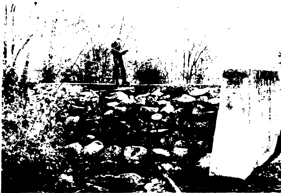
13. Stone facing on downstream side of auxiliary spillway
