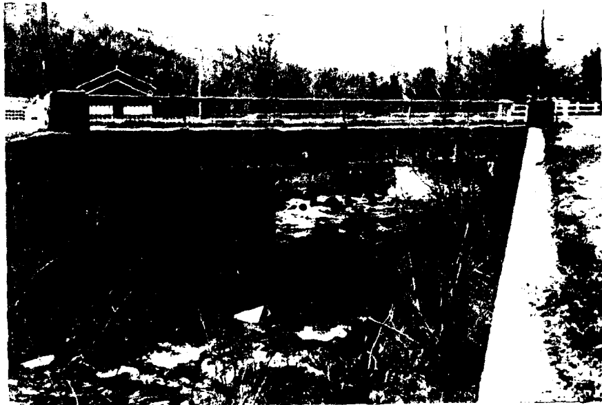
Figure 9 - Concrete bridge at Route 2 in the Village of Charlemont. Note fire station and town garage downstream of bridge to the left in photograph.
