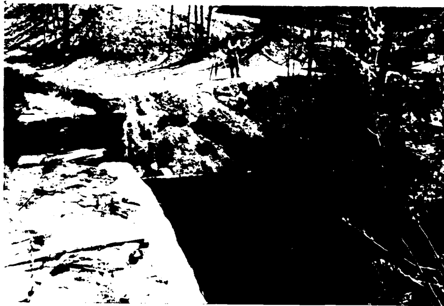
Figure 3 - View of southeast end of dam showing eroded spillway crest, training wall and slope failure at abutment. Note exposed 20 inch water pipe and undermined timber pole retaining wall.
