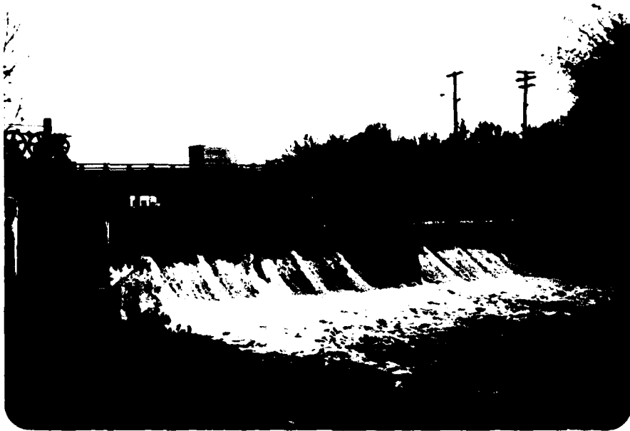
NO. 1 DOWNSTREAM FACE OF DAM
