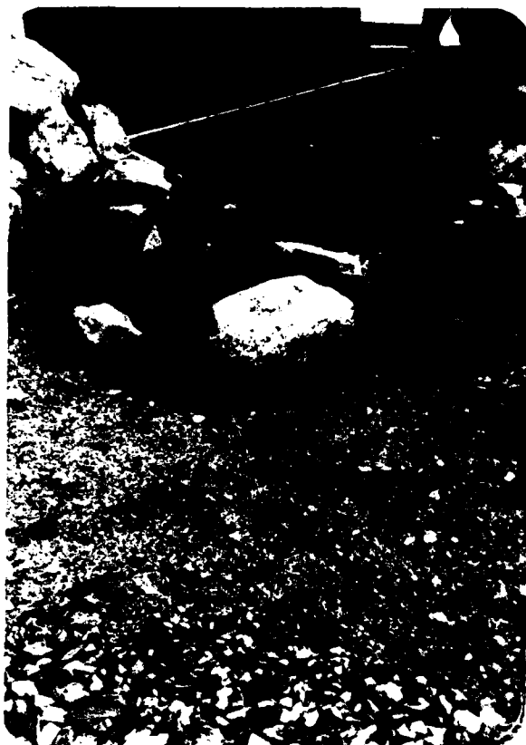
PHOTO NO. 9 - Eroded area on upstream slope of Dam right of the gatehouse as viewed from bottom of slope; scale open to 6 feet.
