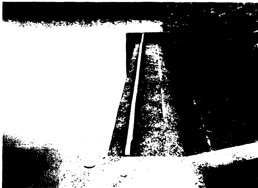
PHOTO NO. 7 - Weir crest and flashboards of the spillway.
