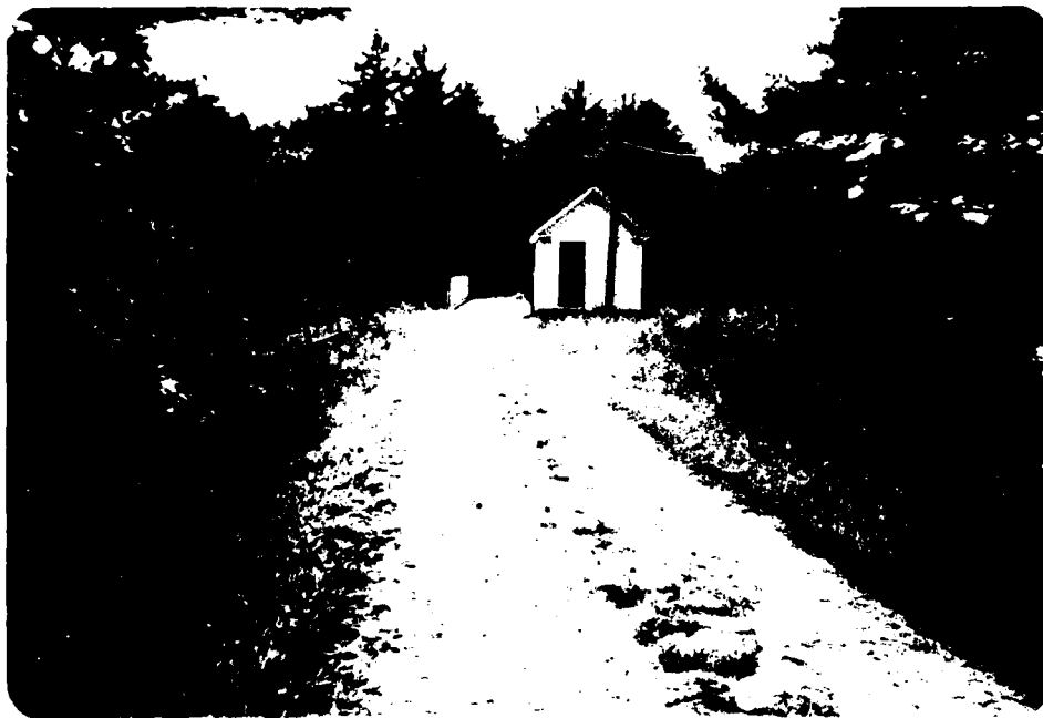
Overview of top of dam from left abutment
