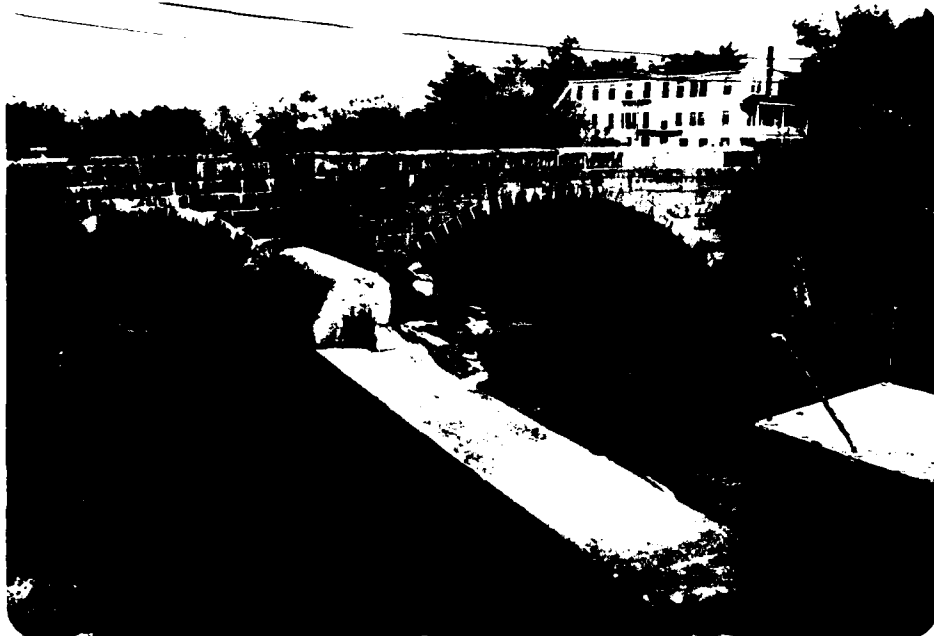
7. View of highway bridge just downstream of dam and of the diversion channel to old mill
