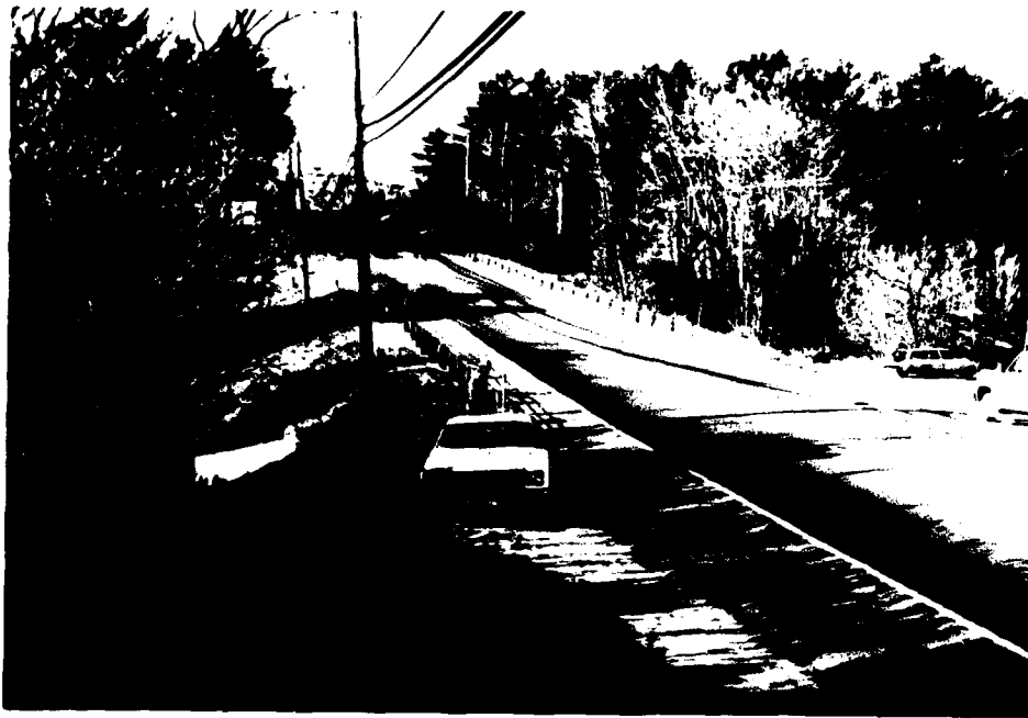
6. Downstream side and alignment of roadway from left end of dam
