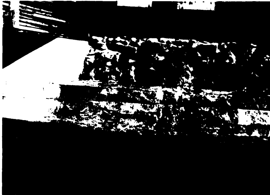
September 18, 1979 Figure 15 - Looking at deteriorated condition of the concrete at the east wall of the downstream channel.
