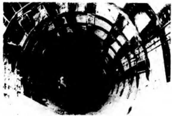
READY FOR LINING
