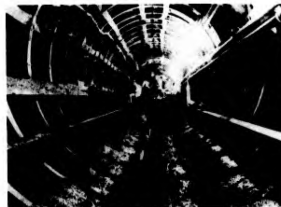
SUBINVERT CONCRETE PLACED TO PROTECT INVERT ROCK
