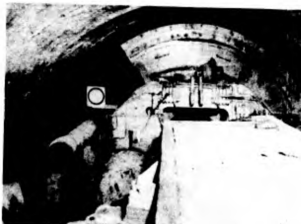
MACHINE AT HEADING. NOTE LASER BEAM TARGET
