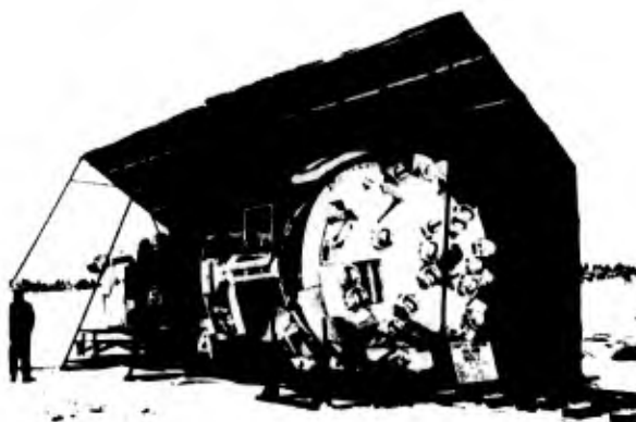
ASSEMBLING BORING MACHINE
