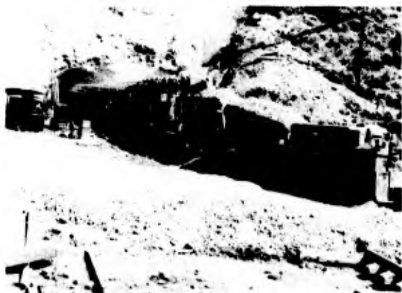
LOADING MUCK CARS AT START OF MACHINE OPERATIONS
