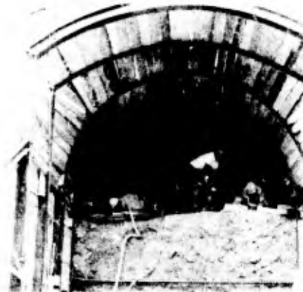
TURNING UNDER AT INLET PORTAL
