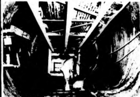
LOOKING UPSTREAM TOWARD HEADING SHOWING 40' BRIDGE SECTION OF MUCK CONVEYOR. THIS PROVIDES SPACE IN WHICH TRACK IS LAYED
