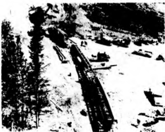
OVERHAULING TUNNELING MACHINE AND BACKUP EQUIPMENT AT OUTLET PORTAL
