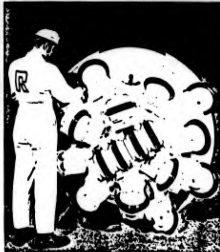
INCLINED BORING MACHINE DIAMETER 6 ft. 1/2 in. (1,84m)
