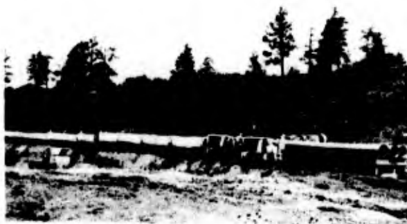
MUCK TRAIN AT DISPOSAL AREA
