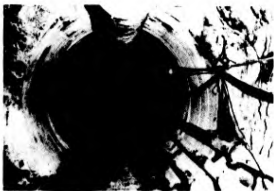
VIEW UPSTREAM AT POINT OF RENEWED MACHINE BORING STA. 397+79
