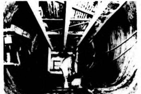
LOOKING UPSTREAM TOWARD HEADING SHOWING 40' BRIDGE SECTION OF MUCK CONVEYOR. THIS PROVIDES SPACE IN WHICH TRACK IS LAYED
