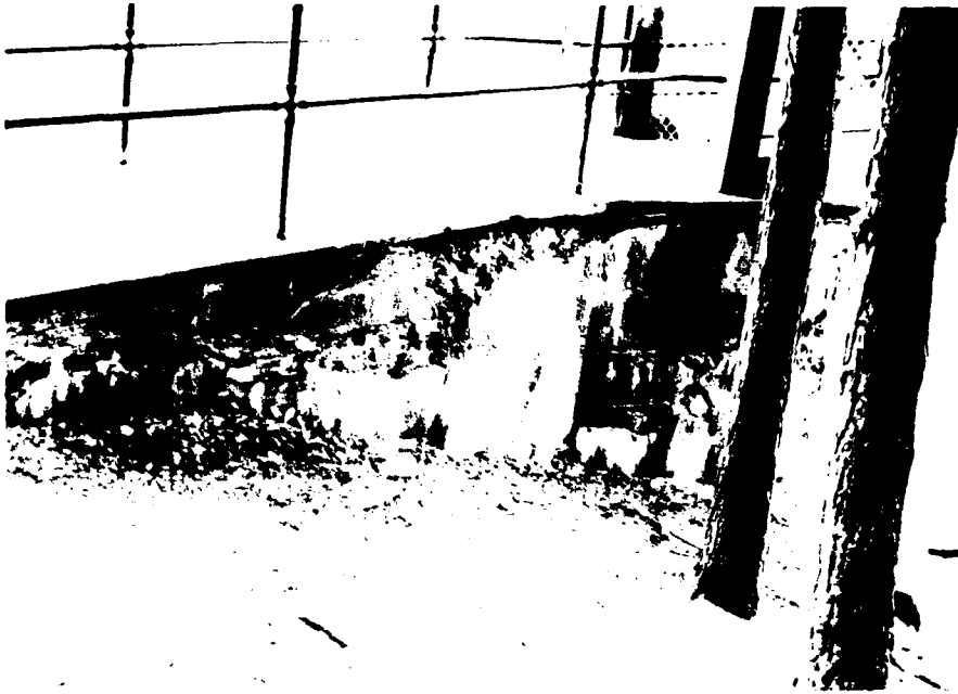
3. Downstream wall of right abutment showing spalling and efflorescence
