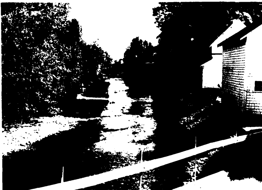
September 19, 1979 Figure 14 - Looking southeast at Reach 4 downstream of Maple Street.
