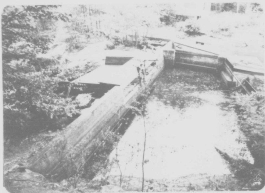
W-1 UPSTREAM FACE OF DAM
