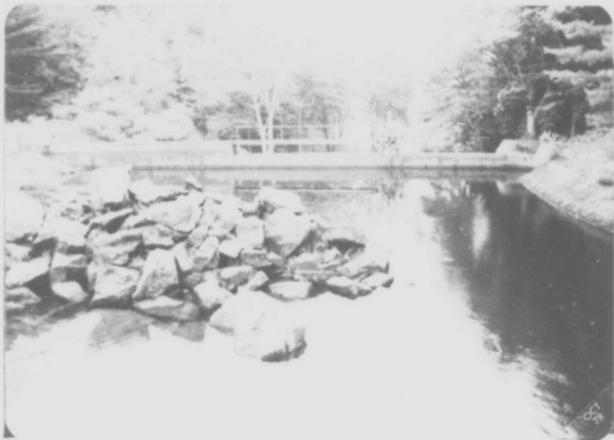
E-2 UPSTREAM FACE OF DAM AND ABANDONED COFFER DAM
