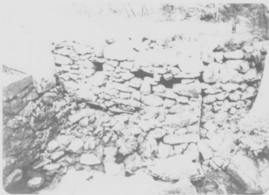
E-8 EMBANKMENT STRUCTURE
