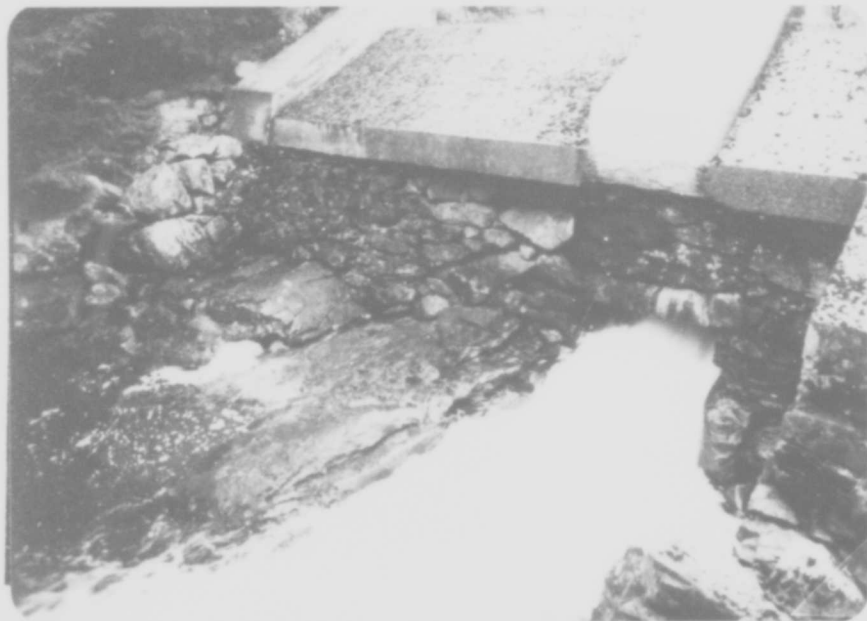
E-1 GATE OPENING AND DOWNSTREAM FACE OF DAM
