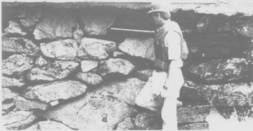
E-9 DOWNSTREAM FACE OF DAM
