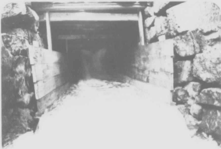
W-4 SLUICWAY OUTLET
