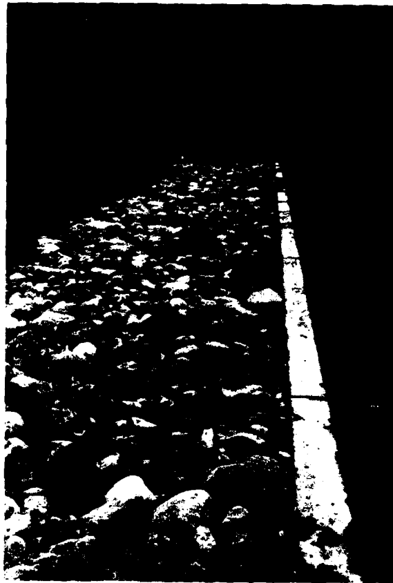
7. View of emergency spillway showing concrete sill with rock rip rap
