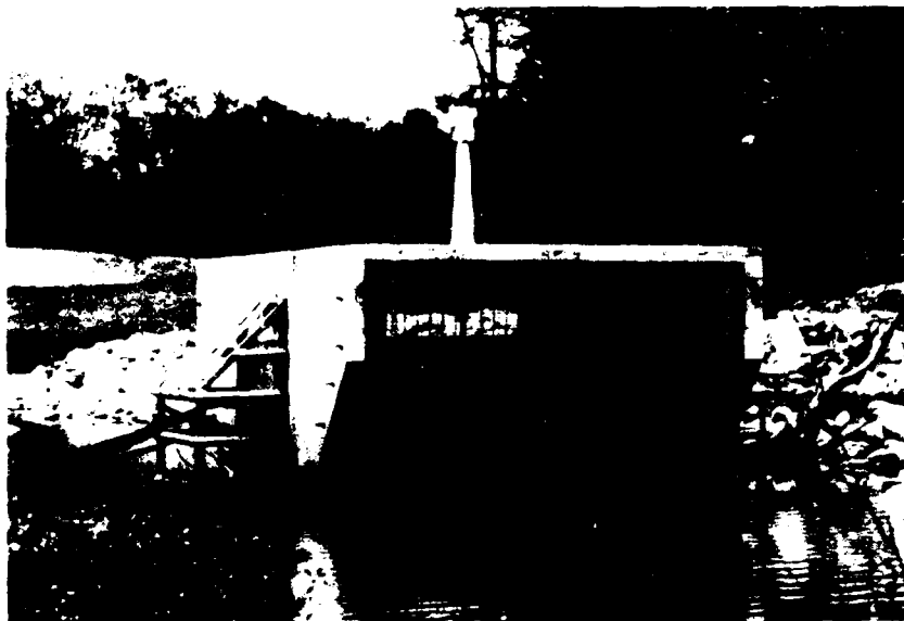
3. View of drop inlet structure showing high and low stage trash racks
