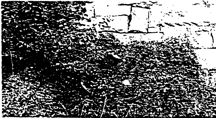
PHOTO #5. Outlet pipe from gatestructure. Note the misalignment of granite blocks beginning to show from heavy growth of vegetation on wall.
