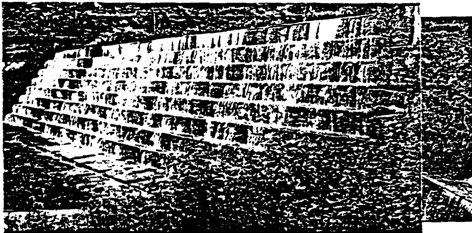
PHOTO #2. Close-up view of stepped masonry face of spillway and stone apron. (UNDER: view across crest also showing heavy growth of weeds. No irregularities noticeable across crest.)
