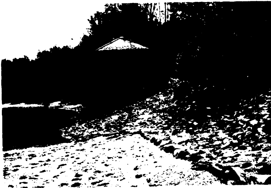
#3 GATEHOUSE AND RIPRAP ON UPSTREAM FACE OF DAM.
