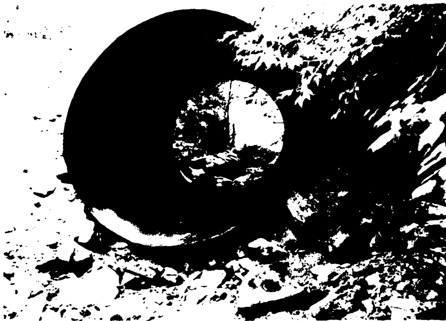
PHOTO NO. 23 - View of downstream end of culvert under roadway.
