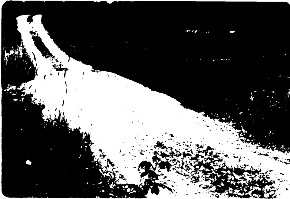
(15) Roadway Across Spillway Channel.
