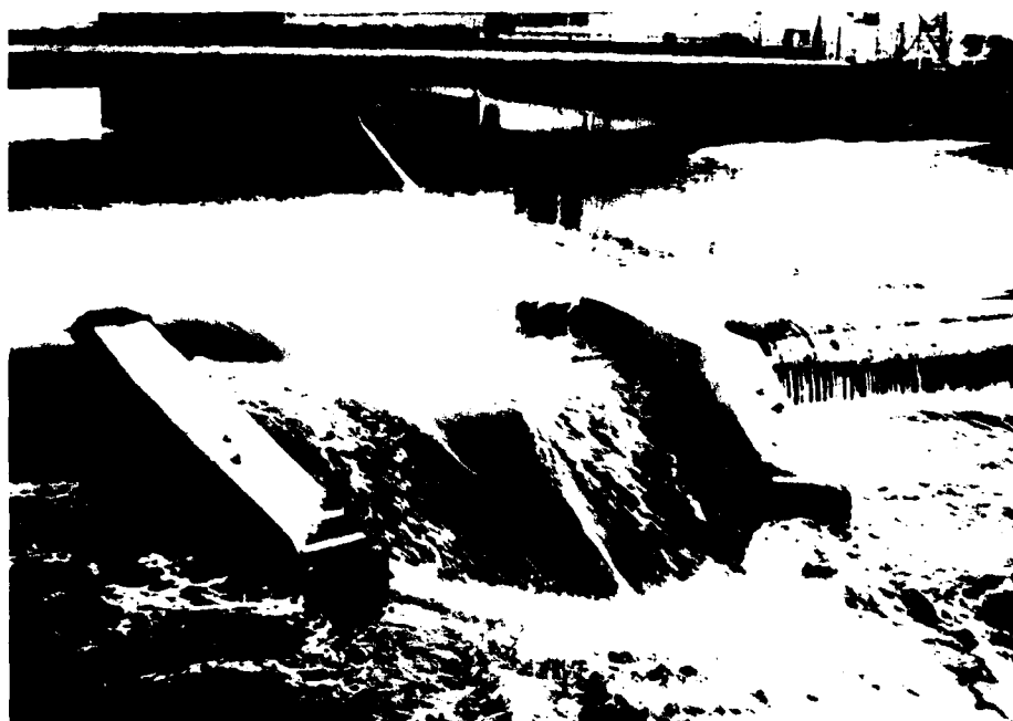
Figure 70. Zuni boat chute, South Platte River, Denver. The rubber fabridam has been modified with a concrete and metal slide to allow passage of canoes and rafts.
