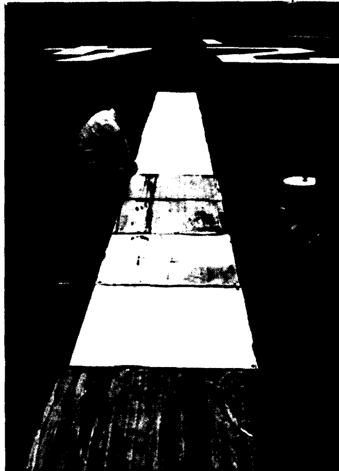
Figure 6. The CAS Tile Marking Line at NAS Miramar (San Diego, California) is Easily Cleaned Despite the Extremely Heavy Rubber Buildup from Aircraft Tires.
