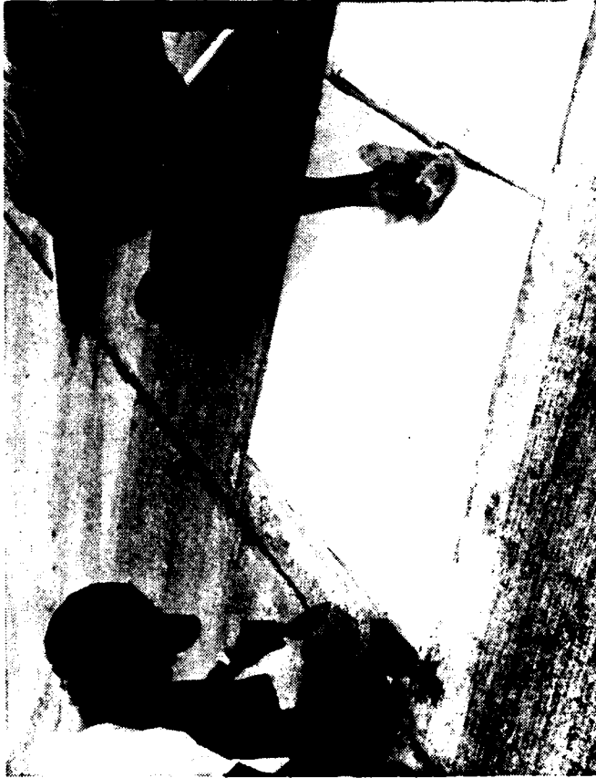
Figure 18. Excess Adhesive is Removed by Wiping with a Clean Rag Dampened (not Soaking) with Methyl Ethyl Ketone Before the Epoxy has Hardened.
