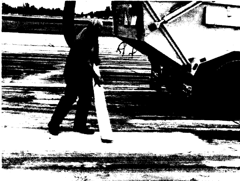
Figure 12. After the Concrete is Ground Down or Planed, the Debris and Water (to Cool the Diamond Cutters) must be Vacuumed off.
