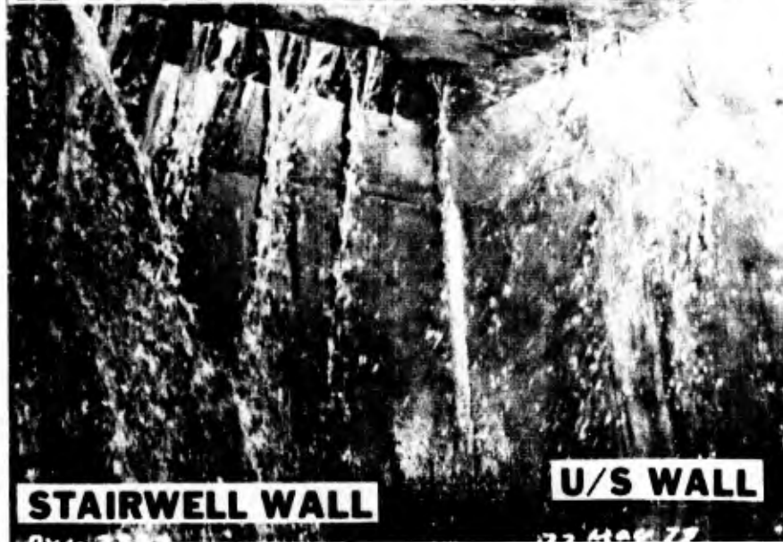
PHOTO #20 EL. 1043 STAIRWELL ROOF
