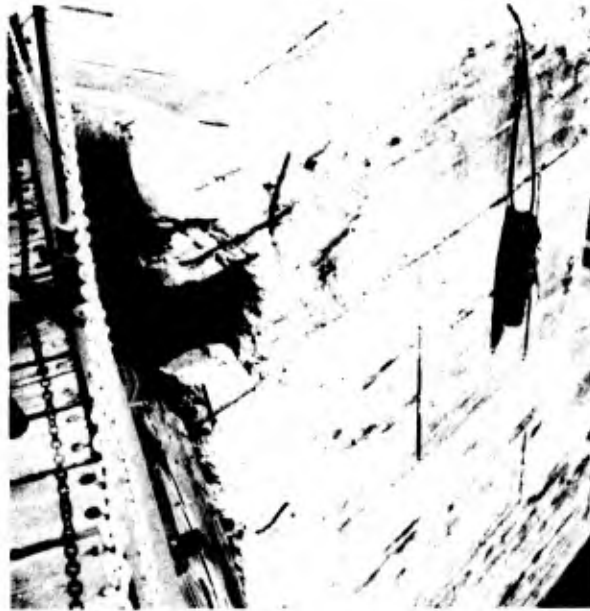
b. Moderate (inadequate concrete cover over reinforcing steel)
