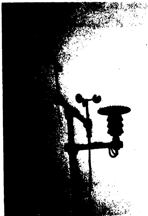
Close-Up of Meteorological Equipment
