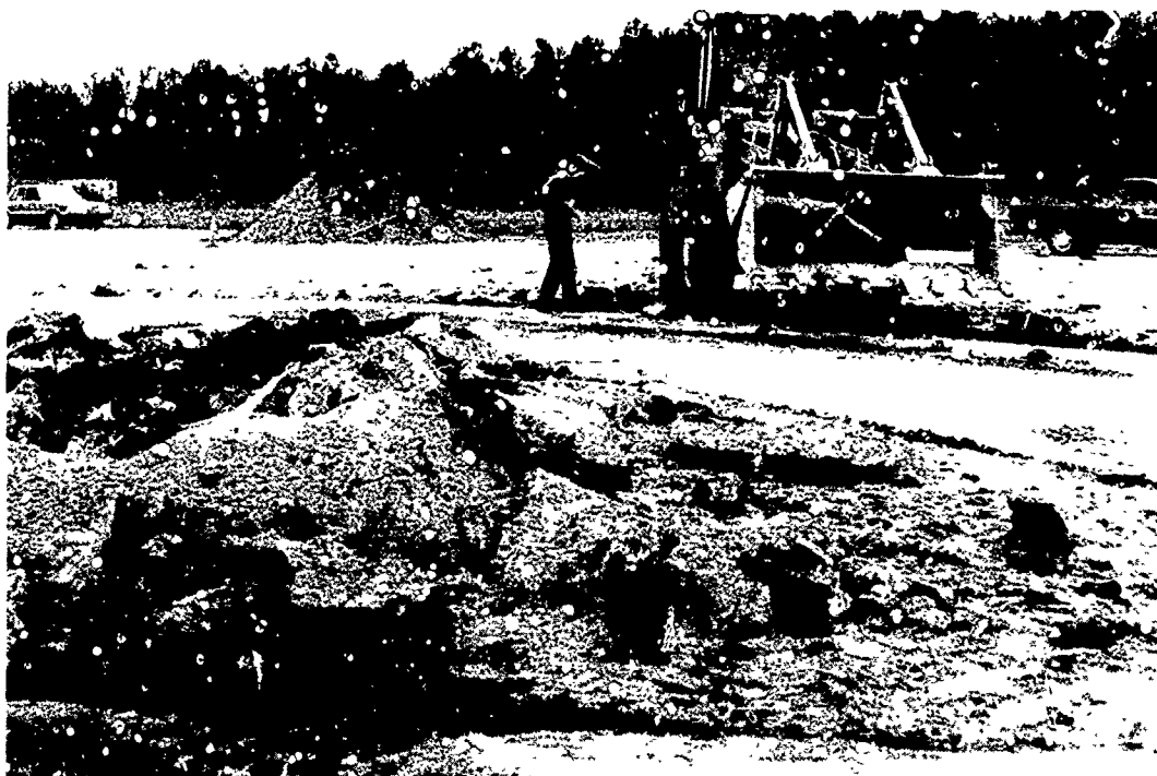
Photo 3. Removing large pieces of debris from precast slab repair crater
