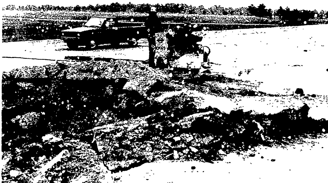
Photo 4. Sawing original PCC to square up precast slab crater
