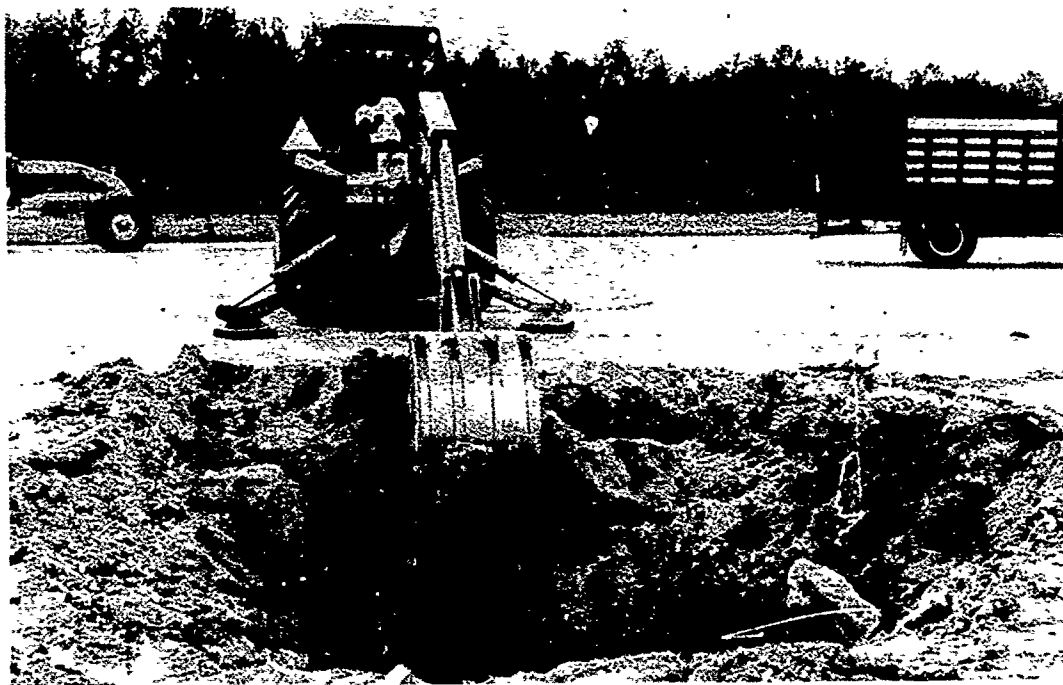
Photo 16. Backhoe pushing ejecta and silty sand into the FOD cover repair
