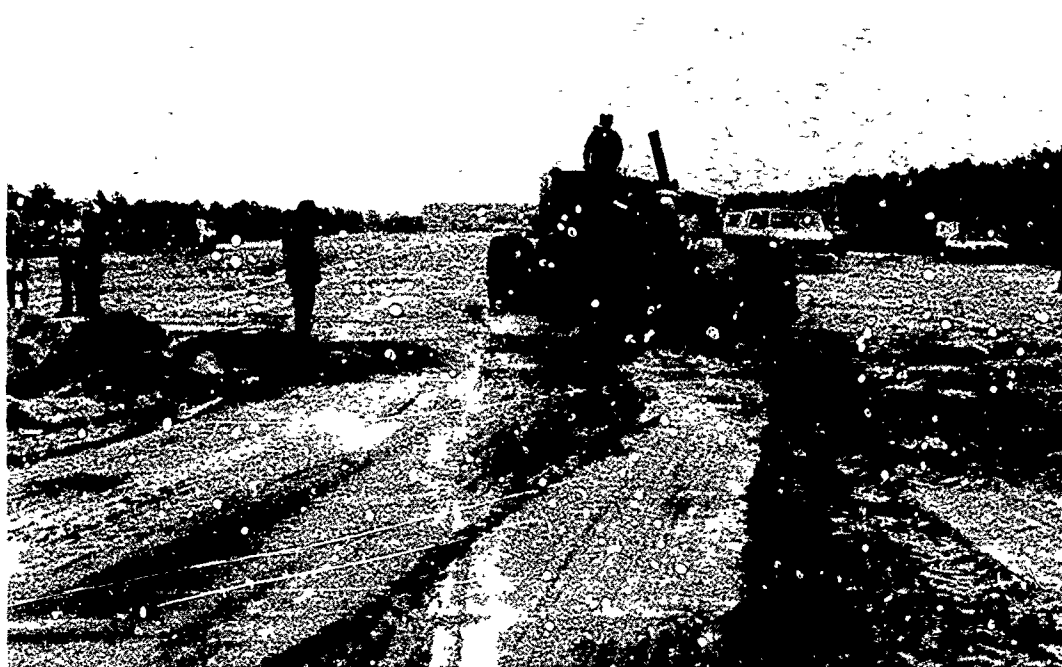
Photo 2. Removing debris from around the crater, precast slab repair
