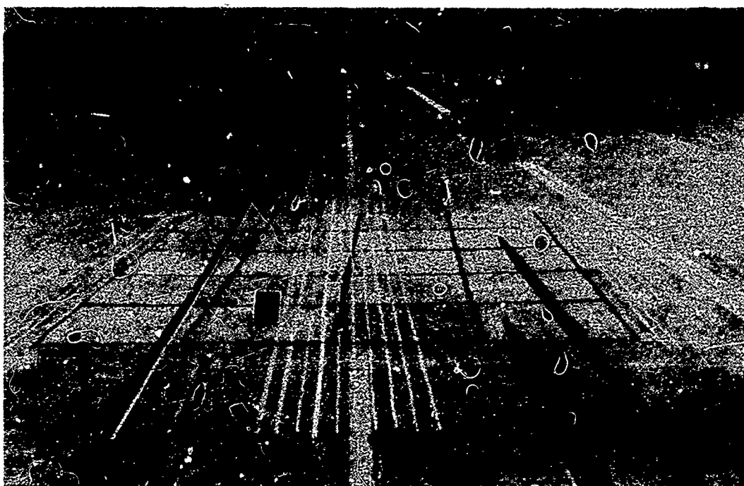
Photo 29. F-15 traffic lane after 2 coverages, precast slab repair
